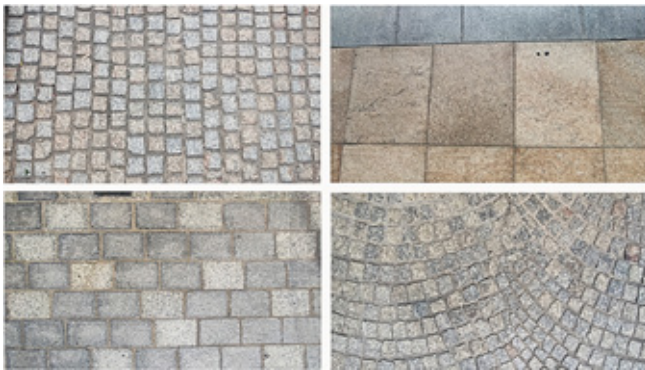
Fig 5. Granite stones and slabs of the actual surface paving in Lithuanian Square, Lublin
