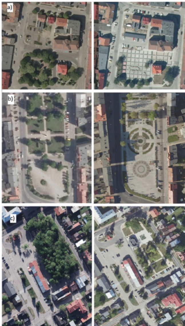
Fig. 2. Exemplary cases of historical parts of cities before and after revitalization: a) Rzepin, b) Kruszewica, c) Janów Podlaski, modified after [22]
