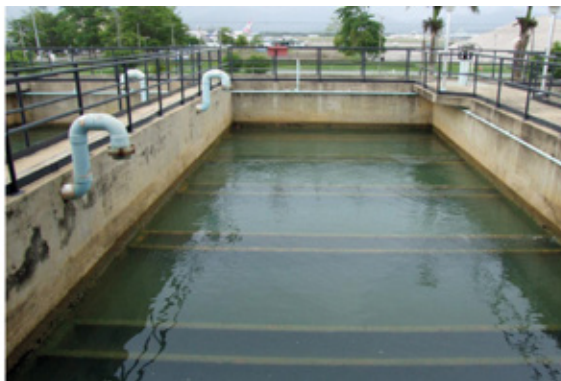
Fig. 1: (a) The Navet Reservoir, Trinidad, West Indies (W.I), with a volumetric capacity of 1.9 million m 3 and area covering 324 hectares of land (b) Secondary Treatment stages of the Caroni Water Treatment Plant, Trinidad, W.I which has a production capacity of 75 million gallons per day. [48]
